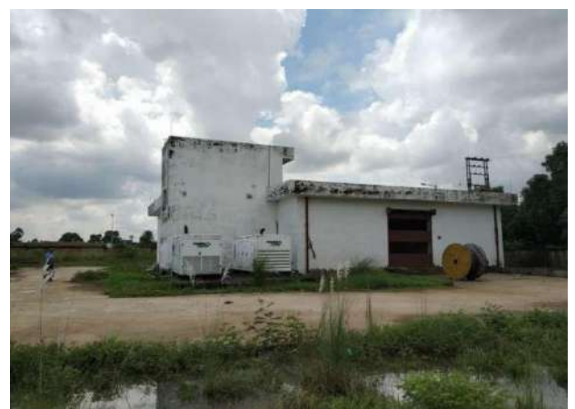
Electric Substation with Power Back UP (DG, 250kVA)
